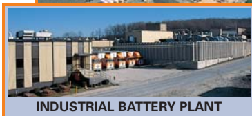
INDUSTRIAL BATTERY PLANT
